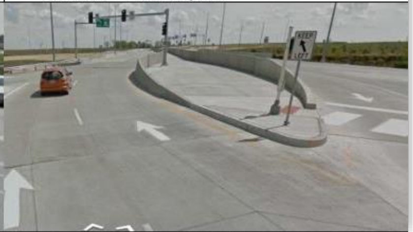
B) Center Walkway, Single Structure Botts Rd. - Branson, MO
