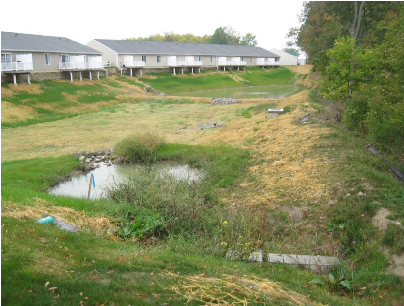
Dry Extended Detention Basin w/Forebay and Micropool
