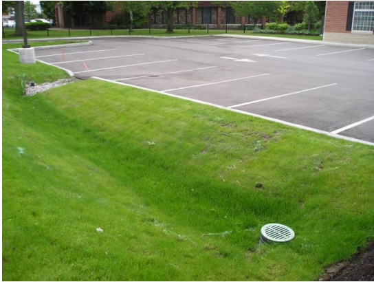
Turfed Linear Bioretention
