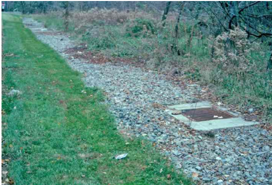
Turfed Linear Bioretention
