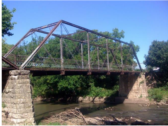
Steel Truss Bridge
